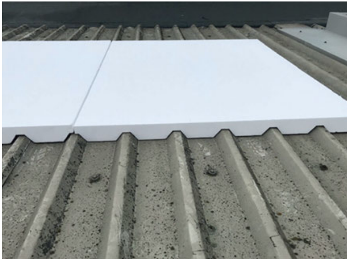
Bespoke EPS insulation cut for existing profiled metal deck.
