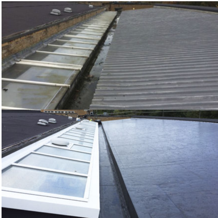
Before and after of profile metal roof overlaid with Bauder Thermofol PVC membrane
