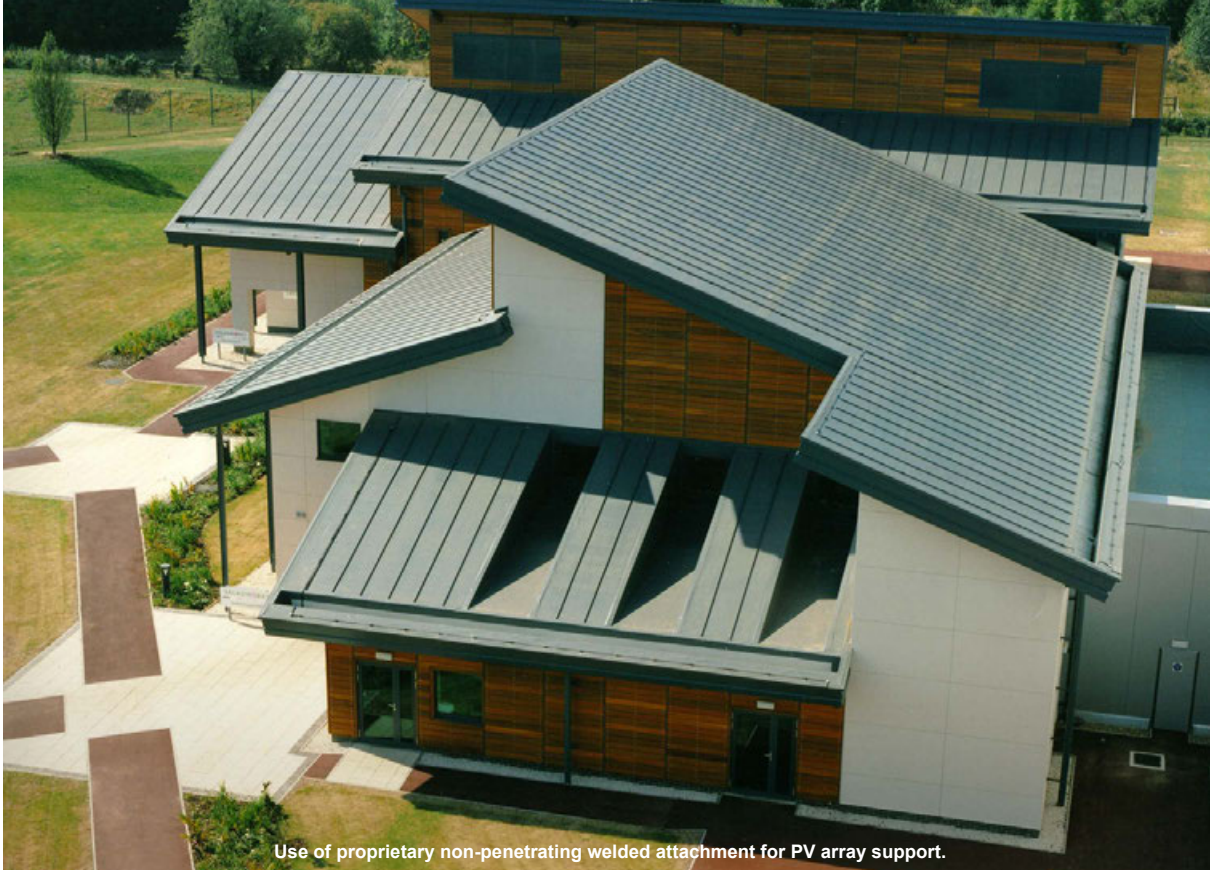
Use of proprietary non-penetrating welded attachment for PV array support.
