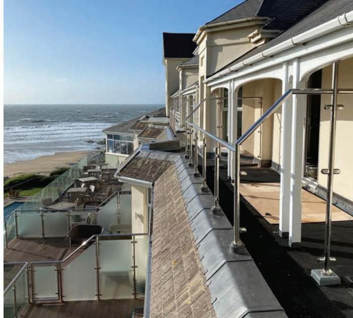
Code 6 lead welted cappings with hidden copper clips on the stunning Watersmeet Hotel terraces in Woolacombe.
