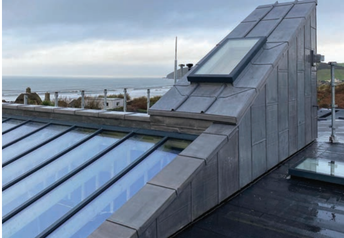
The striking £2million new build in Croyde, North Devon, with its mono-pitch roof completely clad in lead by Zak Williams. The exposed location meant everything was doubly secured, so all free edges were back hooked.
