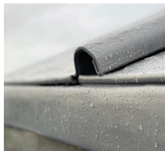
The striking £2million new build in Croyde, North Devon, with its mono-pitch roof completely clad in lead by Zak Williams. The exposed location meant everything was doubly secured, so all free edges were back hooked.
