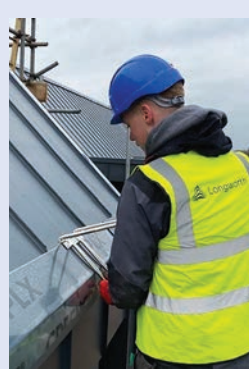
Harry Nibloe, Roofing apprentice Longworth Building Services
