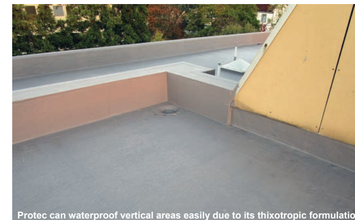
Protec can waterproof vertical areas easily due to its thixotropic formulation.
