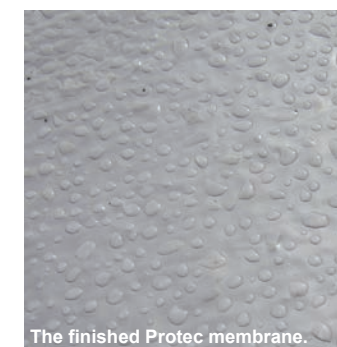
The finished Protec membrane.
