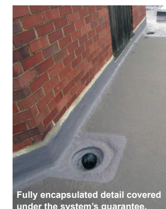
Protec can waterproof vertical areas easily due to its thixotropic formulation.
