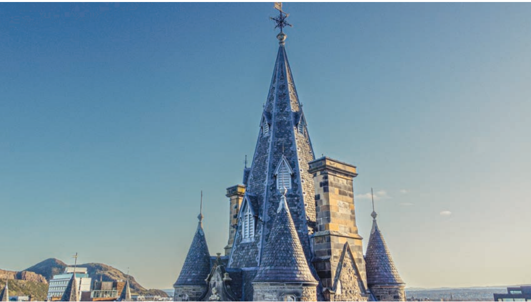
NFRC Scotland Awards 2023 Roof Tiling category winner: Edinburgh Futures Institute: MAC Roofing & Contracting Ltd
