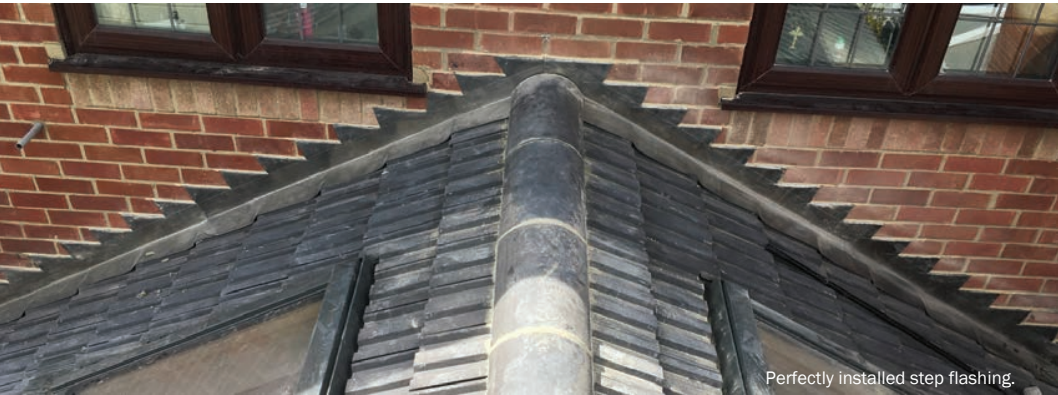
Perfectly installed step flashing.
