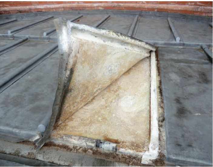
Lead sheet must be laid on a fully and cross ventilated substrate conforming to BS 5250 to avoid underside corrosion.
