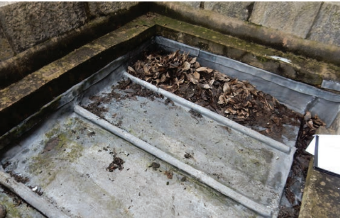
An area of concern was the original, oversized lead gutters to the front, rear and internal elevations. Following an intrusive survey, Hodgson Sayers designed a new lead gutter into specified bay sizes using Code 7 & 8 lead to comply with building regulations.
