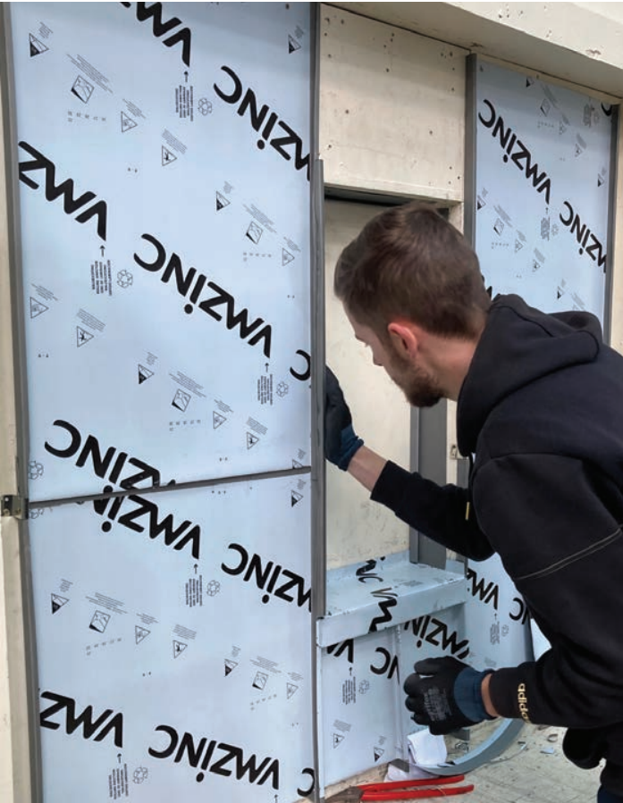
Learning the skills of detailing with hard metals is important to achieve a watertight finish.
