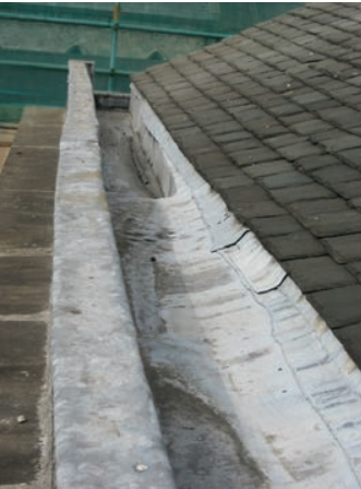
An area of concern was the original, oversized lead gutters to the front, rear and internal elevations. Following an intrusive survey, Hodgson Sayers designed a new lead gutter into specified bay sizes using Code 7 & 8 lead to comply with building regulations.
