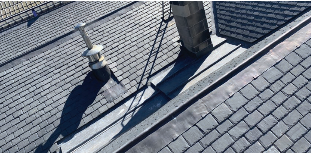
NFRC Scotland Awards 2023 Roof Slating category winner: Sterling Railway Station: John Fulton Plumbing and Roofing
