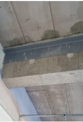
End bearing strengthening.
