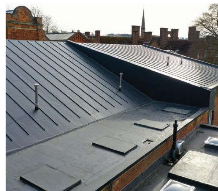
Marlborough College by the Complete Roofing Company Ltd with Bauder Ltd. Winner of Best Detailing 2020 SPRA Award.
