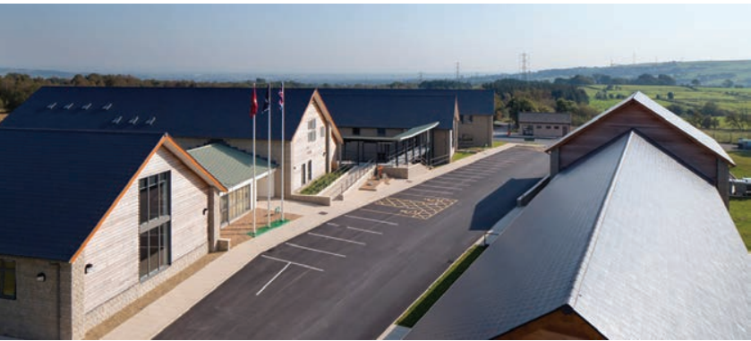
Project 2: With its smooth surfaces and dressed edges, Birkdale has been successfully used with a range of building materials to create series of interlinked buildings for the Greater Manchester Army Cadet Force.
