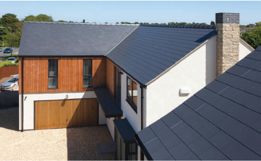
Project 1: The natural textured finish of Thrutone Textured slates perfectly offsets the clean white walls and attractive wood detail on this new build in Grimsby.
