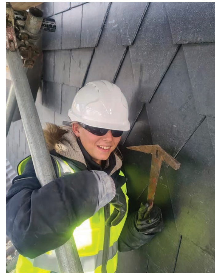
Bobby Mae Smith from G Smith Roofing Ltd, who starts her roofing apprenticeship at Leeds College of Building in the near future.
