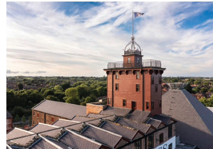
The roof pitch variation between 28° to 63° and the saw tooth design of the main mill were particular challenges in restoring the 1,500m 2 of slate roofs.
