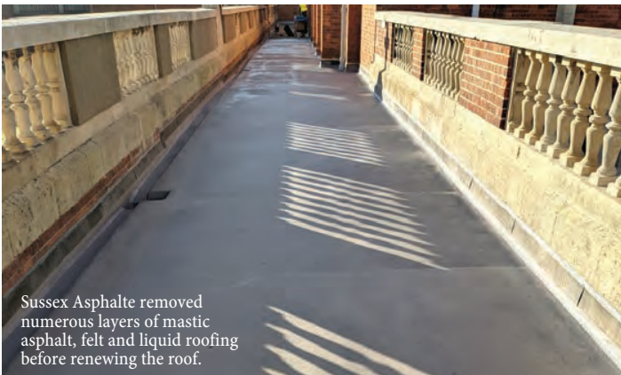
Mastic Asphalt Council (MAC) contractor member, Sussex Asphalte restored the rooftops at Christ's Hospital independent school.
