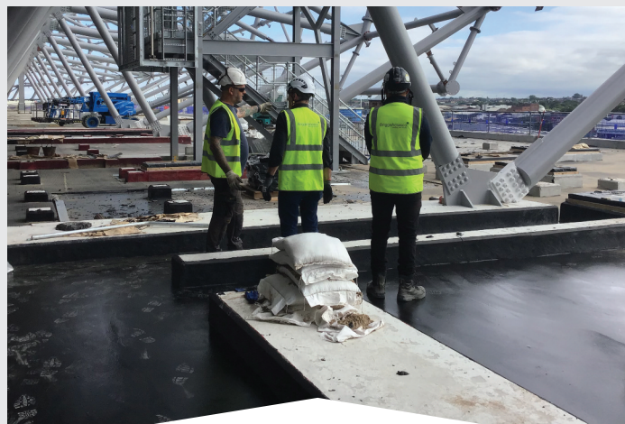
The mastic asphalt roof on the stadium’s east side is well underway. The roof consists of three layers: an isolation layer is laid on the concrete deck before the first 10mm layer of mastic asphalt is applied. A final 10mm top layer is finished with a white, solar-reflective coating to help minimise the roof-temperature and thermal movement across the stadium’s roofs.
