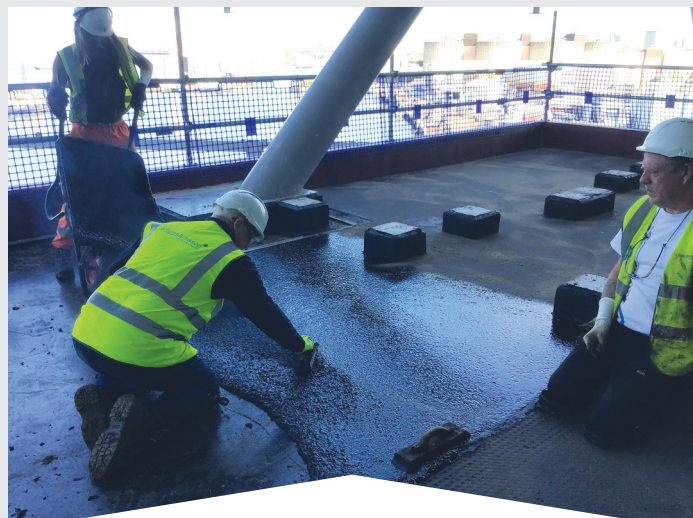
The molten mastic asphalt is wheelbarrowed from the nearby hot boiler to the stadium’s west side roof area where it’s poured. The waiting roofers have to work quickly before the 180°C asphalt cools. It’s a highly-skilled job to ensure the asphalt is laid level, to the correct depth and the joints are watertight.
