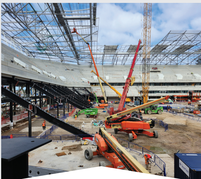
The 13-row concrete seating of the stadium is now in place, covered by a 45m high cantilevered roof structure.
