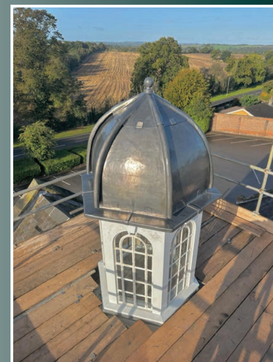
William Simpson at WSJ Leadwork & Roofing completed this striking Code 6 hollow roll cupola at a pub restaurant near Dudley.
