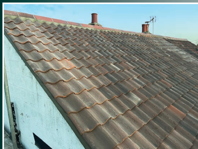
Joe Turner from J3 Roofing & Facades completed a re-roof of this 1712 cottage. The original pantiles were past saving and so were replaced with William Blyth Light Antique Barco Old English pantiles, seamlessly combining with the adjoining property's roof. The ridge tiles were reused, following the less than straight line of the 300+-year-old roof timbers!
