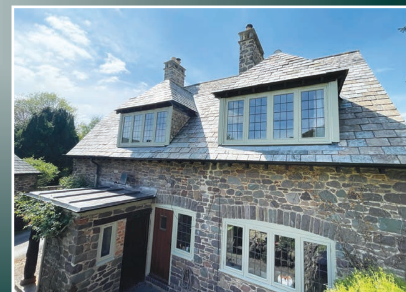
Devon-based Nathan Spice Roofing and Leadwork skillfully achieved this stunning re-roof of a Grade II listed property in Porlock using random diminishing reclaimed Delabole slate.
