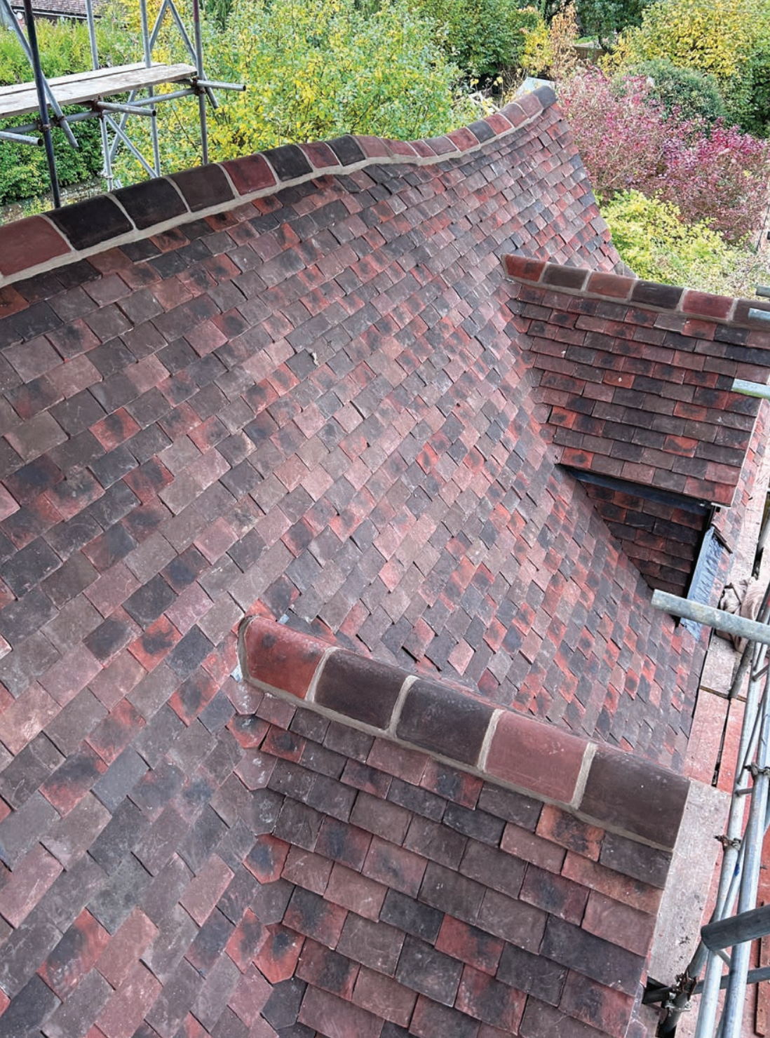
ABOVE: Handmade plain tile roof with handmade clay ridge tiles bedded on NHL mortar by Dean Aston, Aston Roofing.
