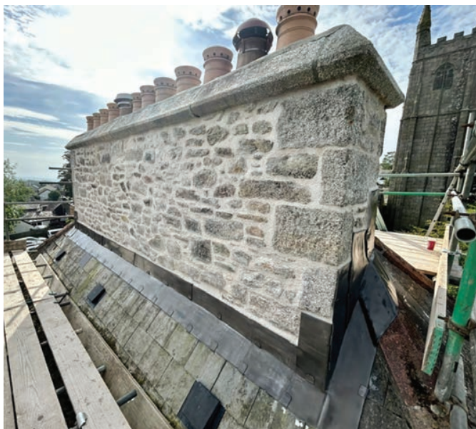
ABOVE: Handmade plain tile roof with handmade clay ridge tiles bedded on NHL mortar by Dean Aston, Aston Roofing.
