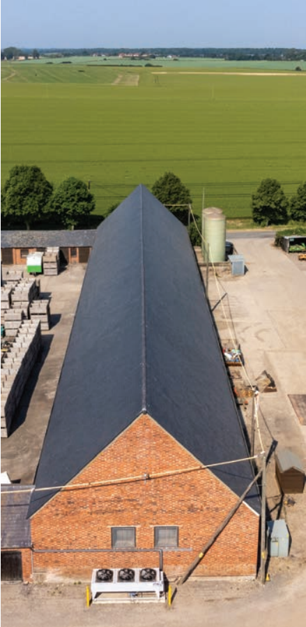
PICTURED - the Grade II listed Chislet Barn reroofed with 500x250mm Gallegas 39 from the SIGA Excellence range of Natural Slate.
