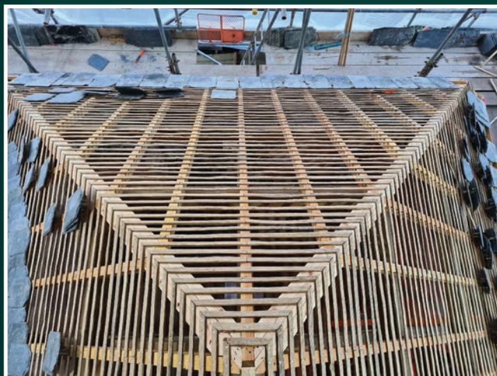
The beauty and skill of a perfectly calculated and setout batted roof! This one was prepared by Heritage Roofing Southwest Ltd, Devon prior to slating the Domesday Barn roof.
