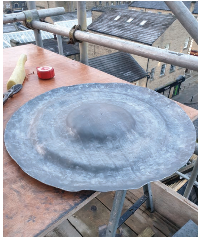
An example of 'waves' being formed to move material from the outside of the lead sheet to the middle area. In this instance a ball was to be bossed in Code 5 lead.
