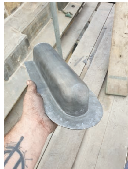
Code 5 cap end detail bossed for a king roll style junction.
