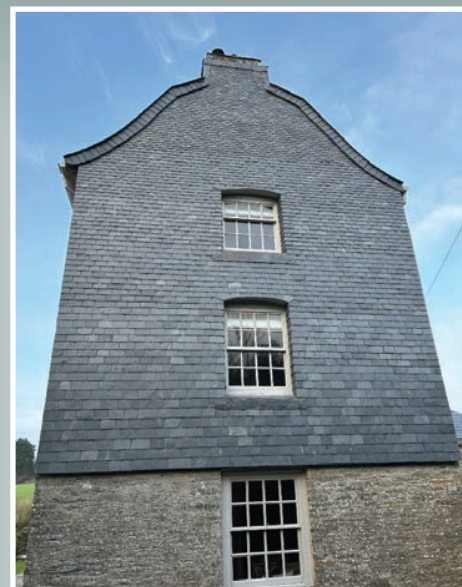
This beautifully slate clad three-storey house in Kingsbridge, Devon was expertly executed by Russell Blackaller of Heritage Roofing Southwest Ltd.
