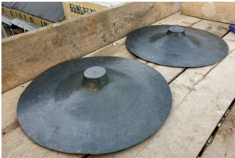
Code 6 bossed discs to weather ornate finial detail.
