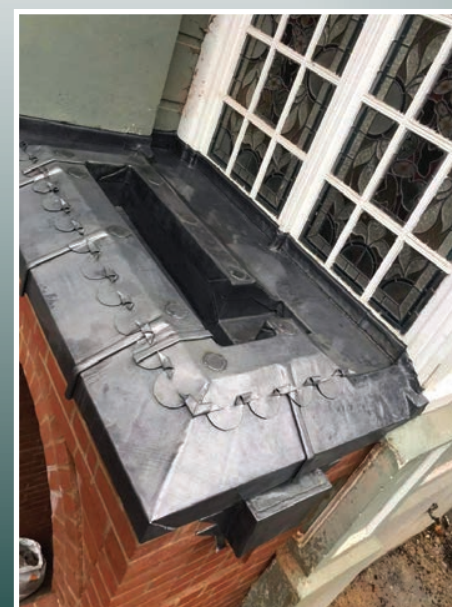
This superbly skilled lead detail was accomplished by Sam Hallett working on a private residence in Reading for main contractor JH Roofing Ltd.
