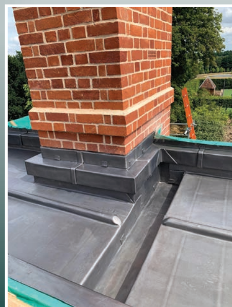
A Code 7 lead roof with Nicholson airtrak ventilation expertly assembled by Ben Nunn of Paul Nunn Roofing Ltd.
