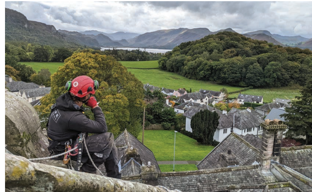
Highlife Rope Access Director, William Oates enjoying the view over the Lake District during a church rooftop inspection.
