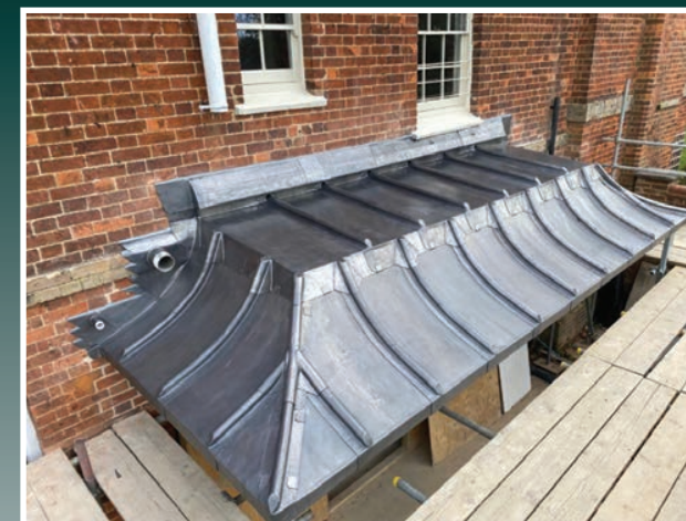
This curved lead conservatory roof on the Old Vicarage, in a Hertfordshire village was superbly crafted in Code 5 lead sheet with a vented drip and vented cover flashing by WJS Leadwork working for MDP Building Services Ltd.
